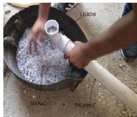
b) Ionic conductor's preparation.
