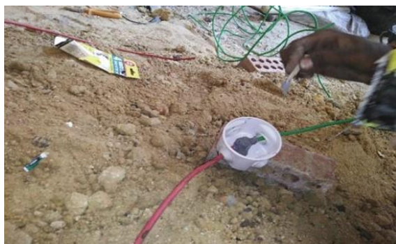
Fig. (13): Splice kit for cables connections.
