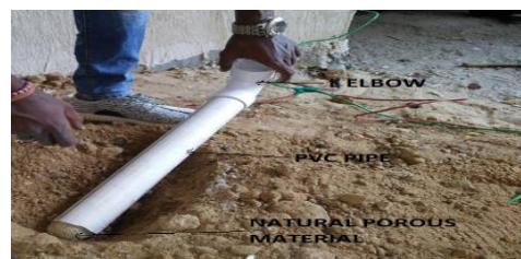
c) Ionic conductor's installation.
