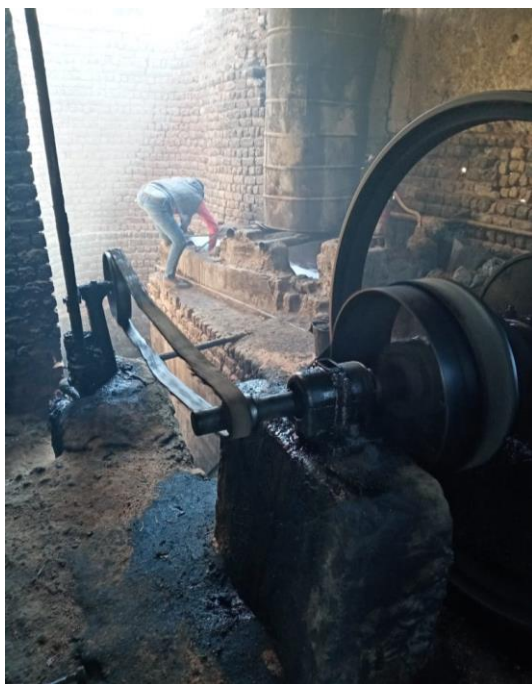
Fig. 3. Photo showing the leakage of petroleum derivatives.
