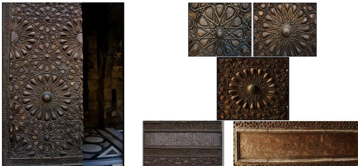
Fig.25. Details of the access door on the eastern facade of the Barquq Mosque [43]
